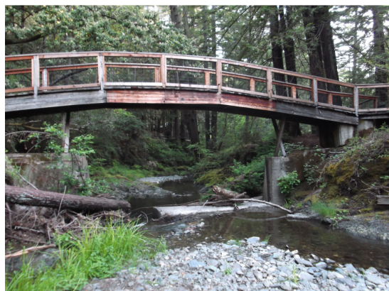
Dam Used to Be Under Footbridge
