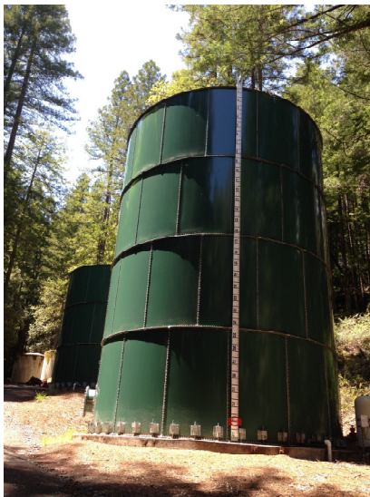
Water Storage Tanks
