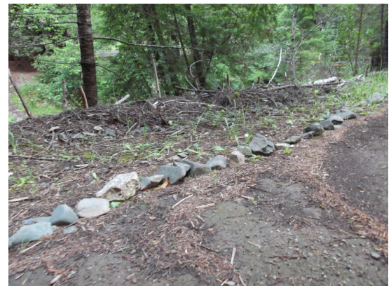
Check Dam beyond Rock-Lined Path
